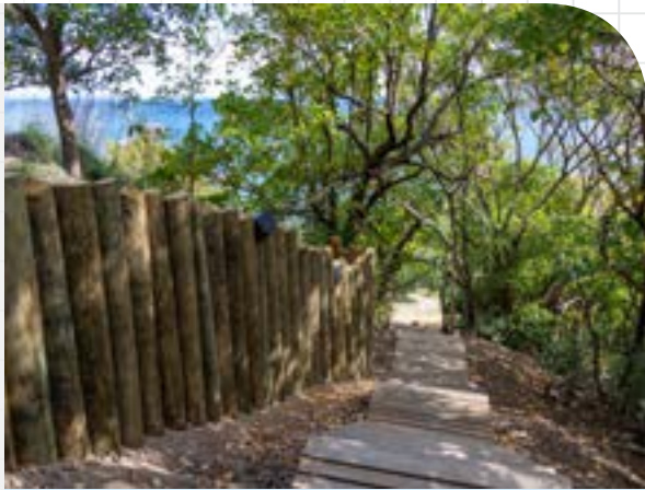
New Pigeon Island Trail in construction stage
