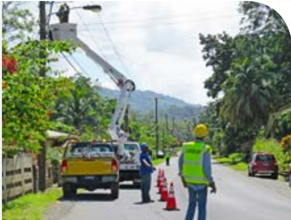
Street light maintenance
